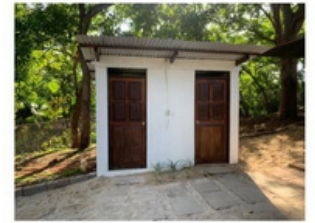
NOW - Renovated Bathrooms
